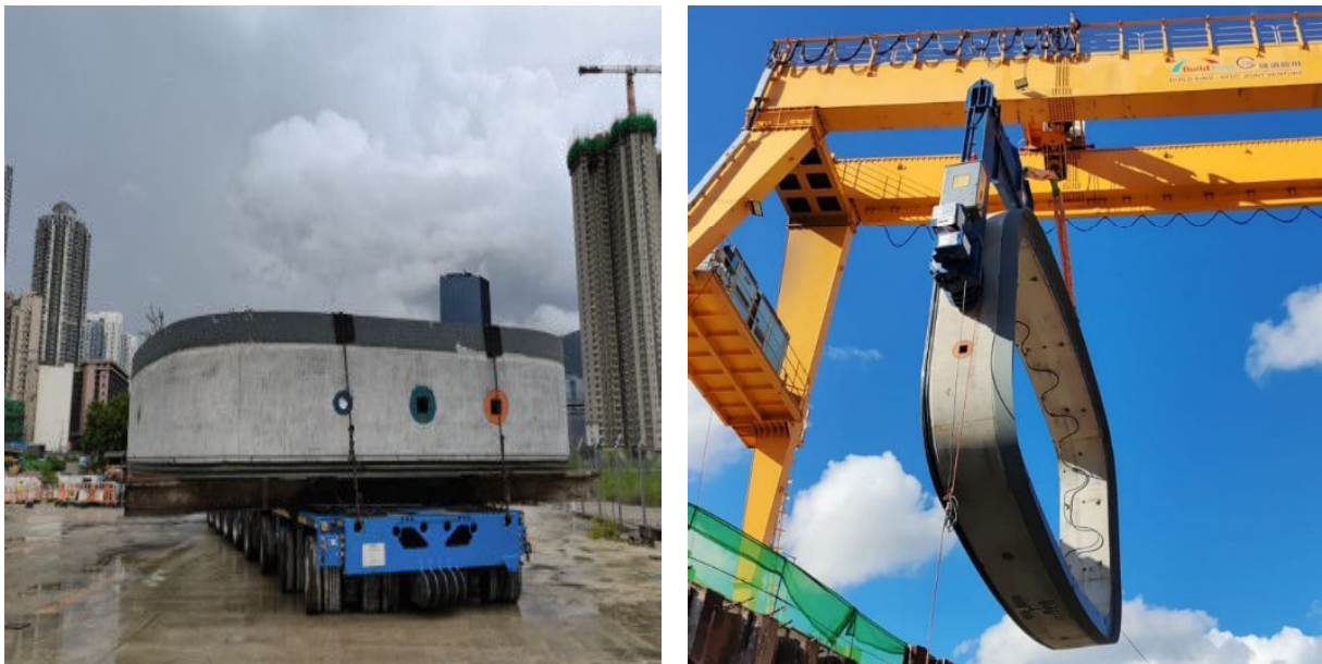
Figure 20 - Transport Tunnel Segment by using Remote Controlled SPMT and Lifting Operation by 115 Tonnes Gantry Crane
