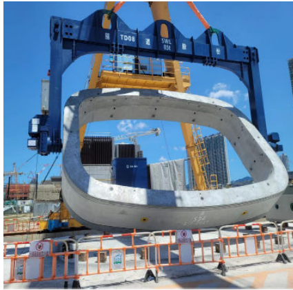
Figure 21 - Newly developed Turning Device for Turning Tunnel Segments upright for Subsequent Installation into Launching Shaft
